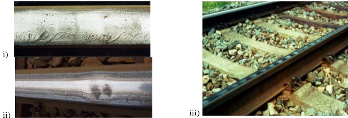
**Figure 2.** An example of i)headcheck failure, ii)undulation defect and iii)scour defect.
